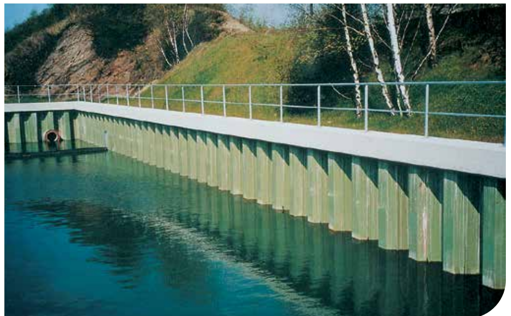
Stormwater retention basin, Lübeck, Germany
