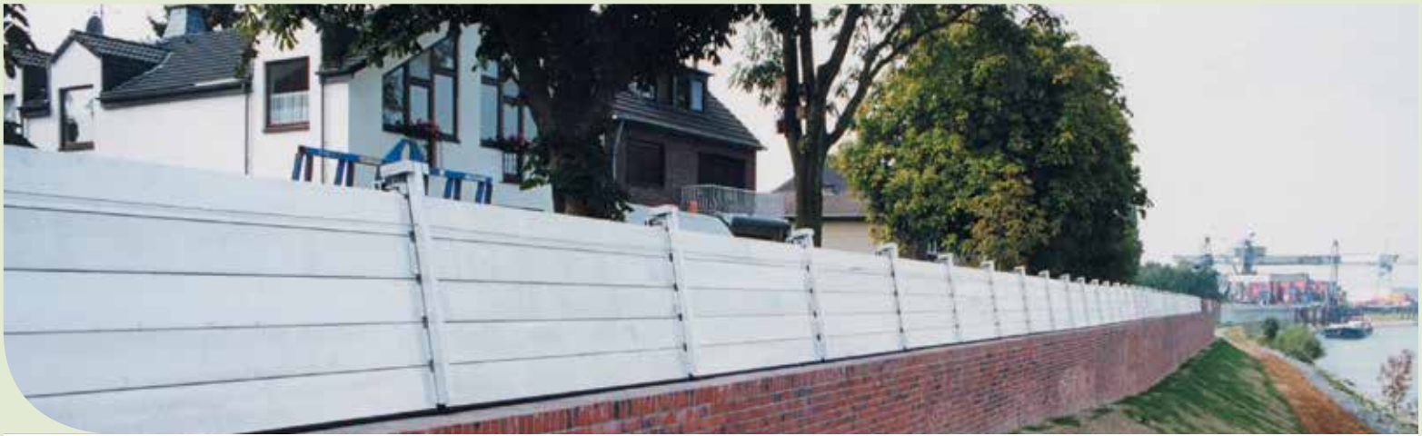
Raising of an embankment in Zons (Germany) – removable panels used for temporarily raising the protection level above the permanent flood-protection level
