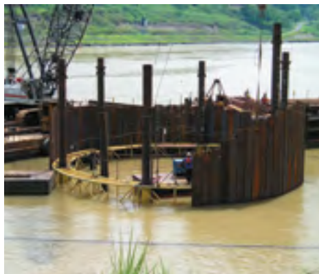
2. Threading until cell closure
