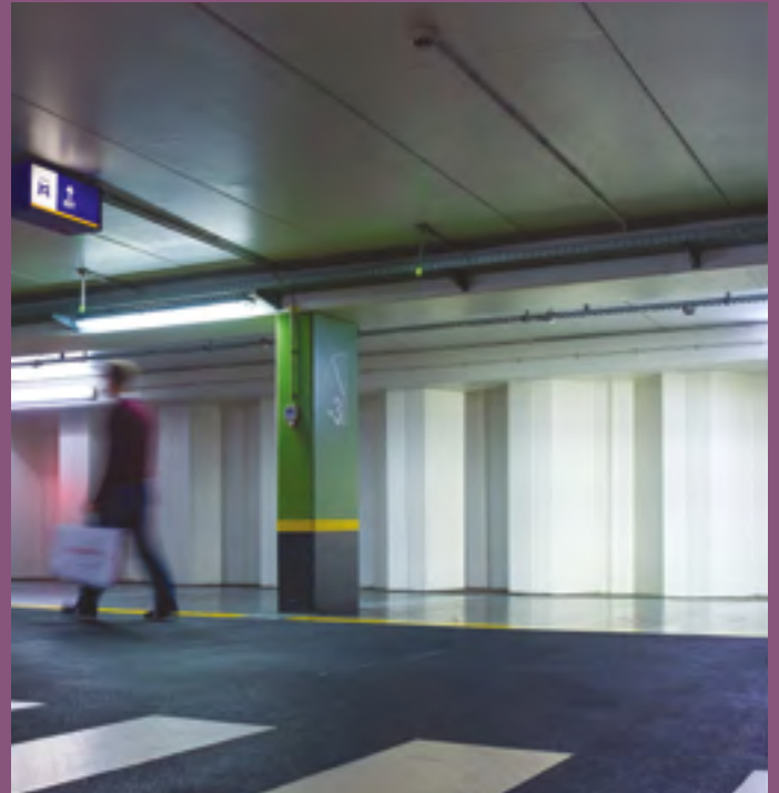
Underground car park with permanent steel sheet pile walls at Hopmarkt shopping center, Aalst, Belgium
