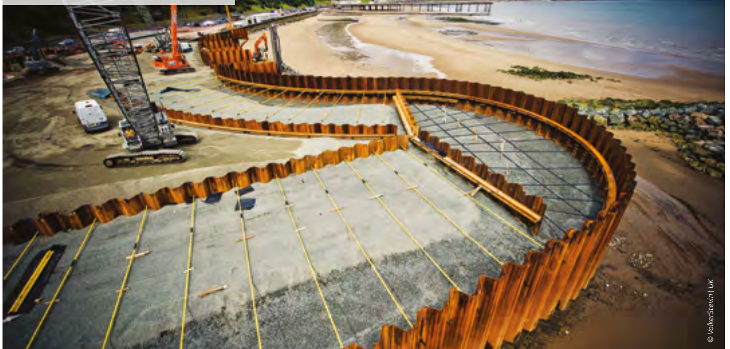
Coastal defense project, Colwyn Bay, UK
