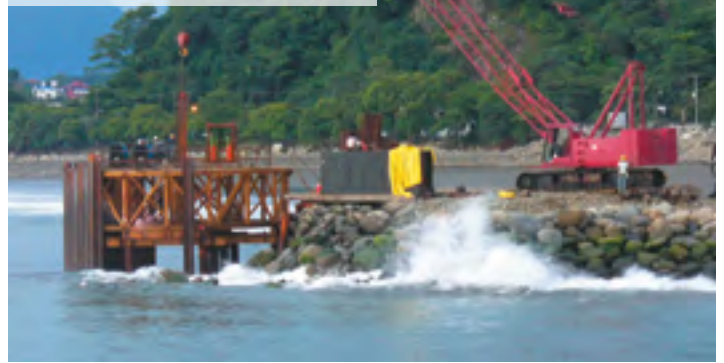
Marina breakwater, Costa Rica
