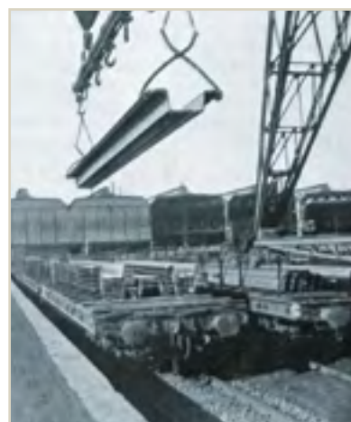
Belval steel works, Luxembourg, 1930s
