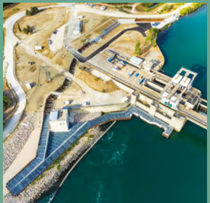
Fish pass at Sauveterre hydroelectric dam on river Rhône, France, allowing the restoration of the migration path of several fish and wildlife species. © Juan Robert
