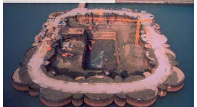
Bridge construction, South Korea
