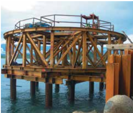
1. Installation of template
