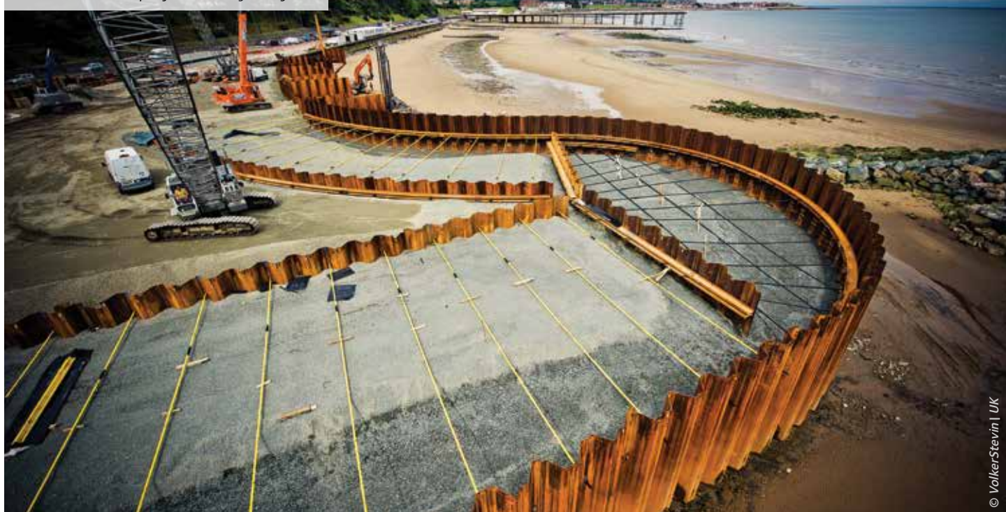
Coastal defense project, Colwyn Bay, UK
