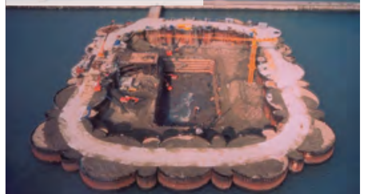
Bridge construction, South Korea
