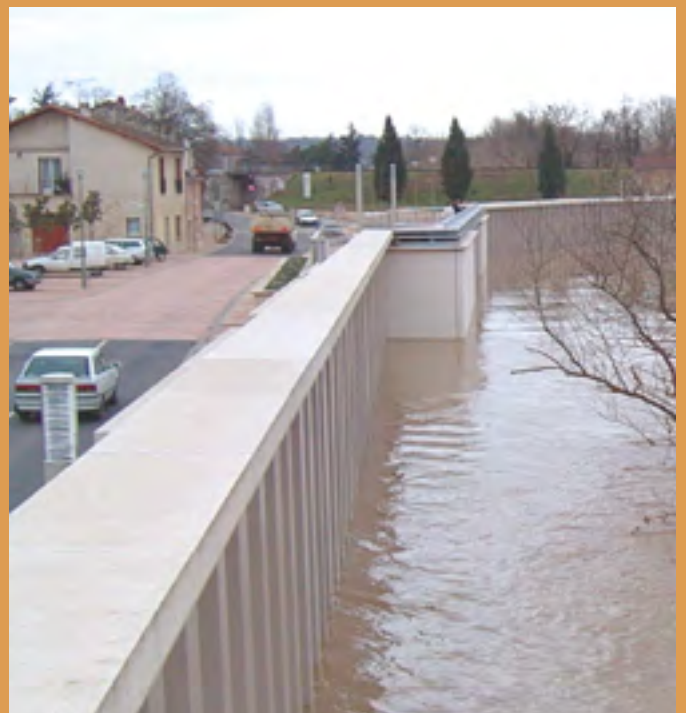
Flood protection barrier protecting the city of St-Pierre de Gaubert, France
