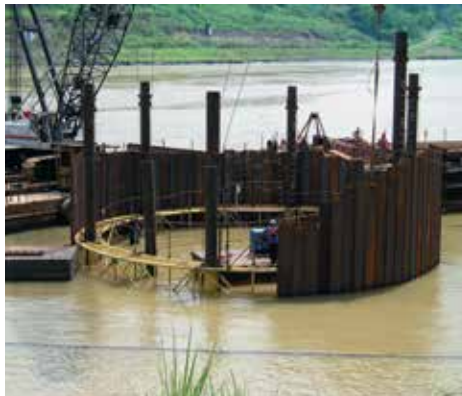
2. Threading until cell closure
