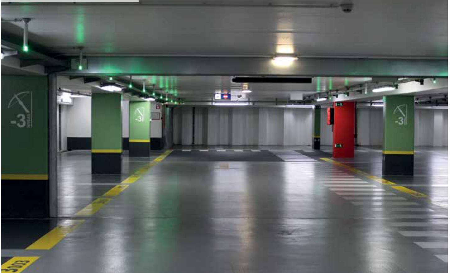
Underground car park, Aalst, Belgium
