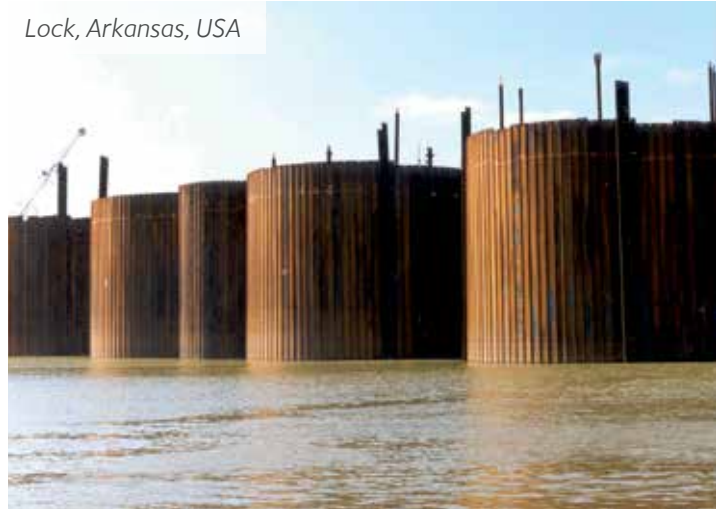
Diaphragm cells with 120^\circ junction piles.
