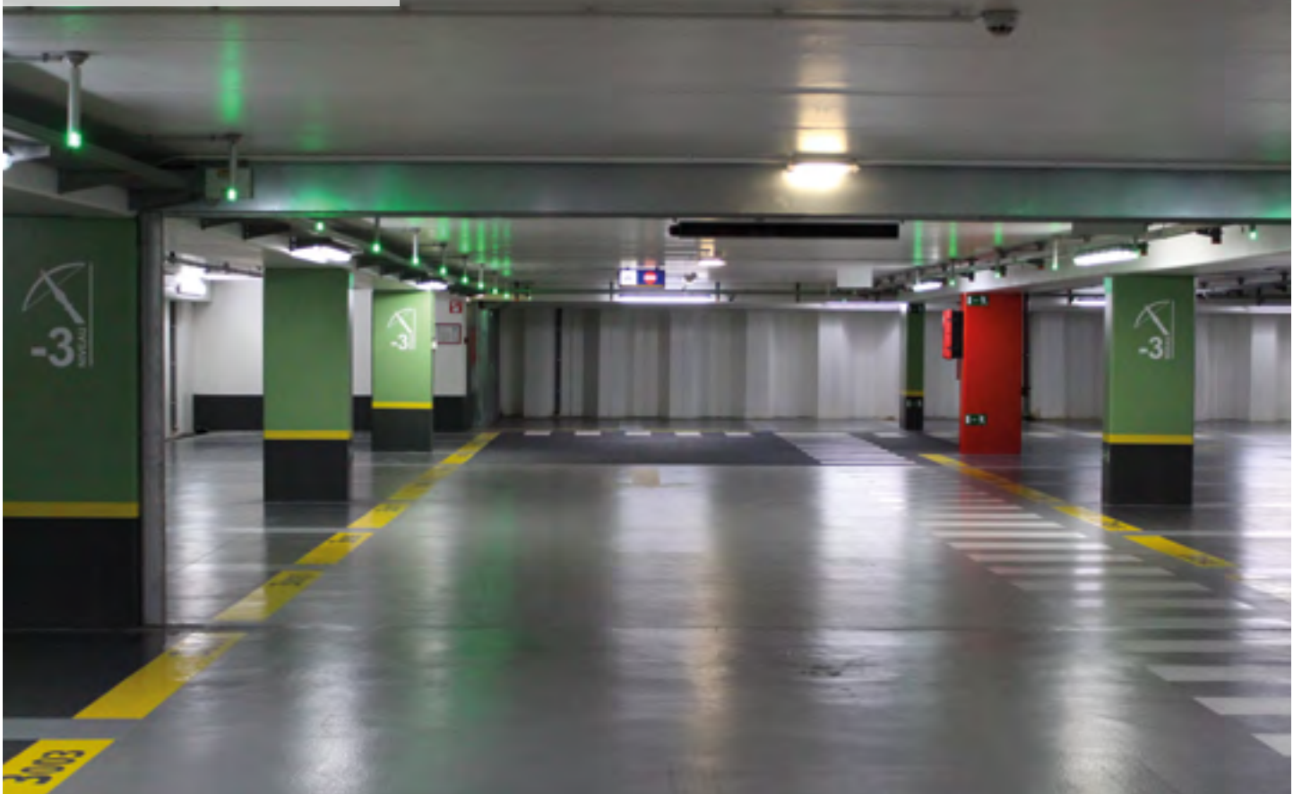
Underground car park, Aalst, Belgium
