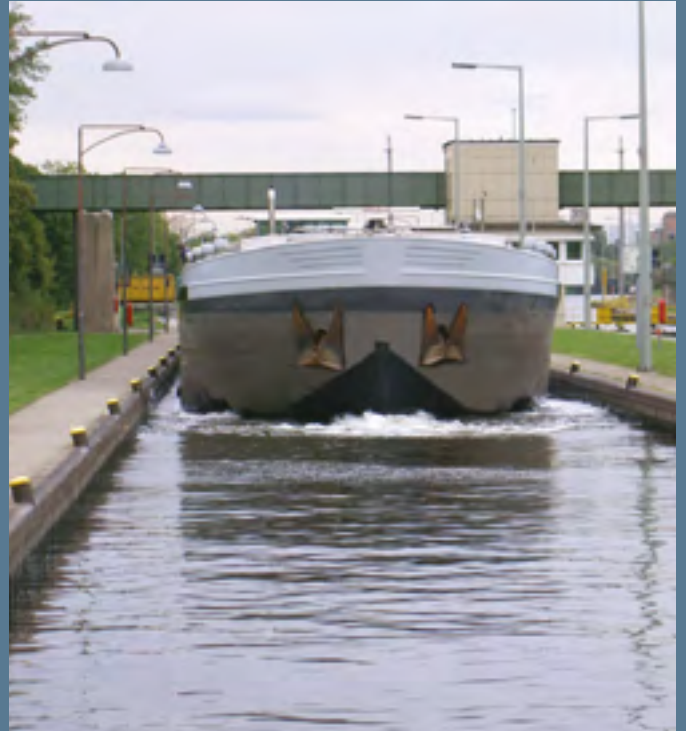
Ship lock on river Main at Eddersheim, Germany
