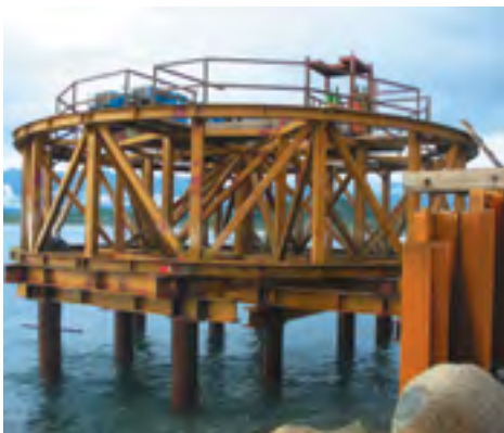
1. Installation of template
