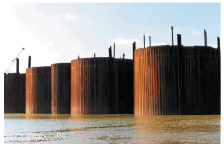
Diaphragm cells with 120^\circ junction piles.
