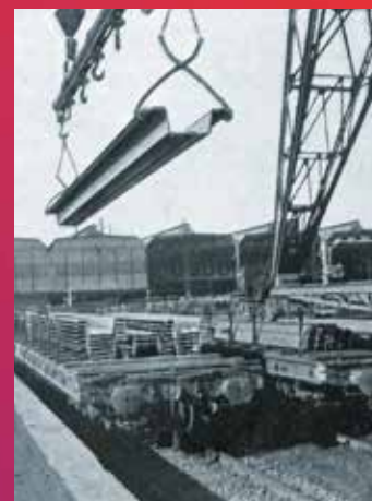
Belval steel works, Luxembourg, 1930s
