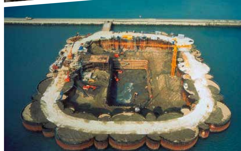
Bridge construction, South Korea
