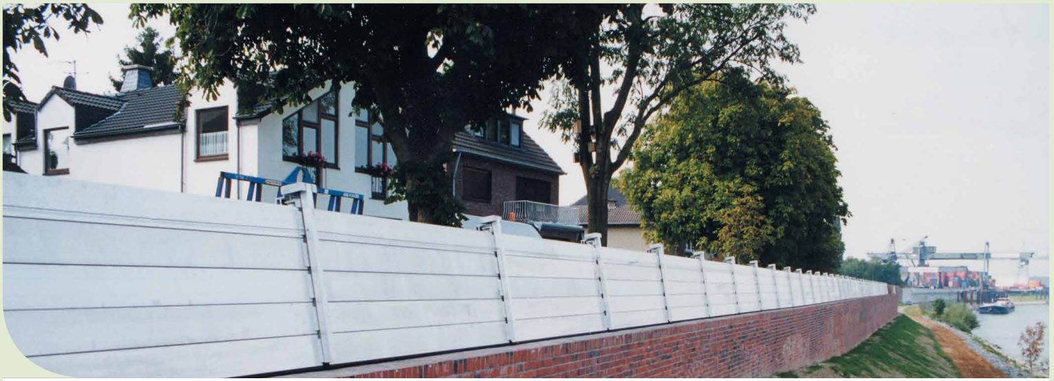
Raising of an embankment in Zons (Germany) – removable panels used for temporarily raising the protection level above the permanent flood-protection level
