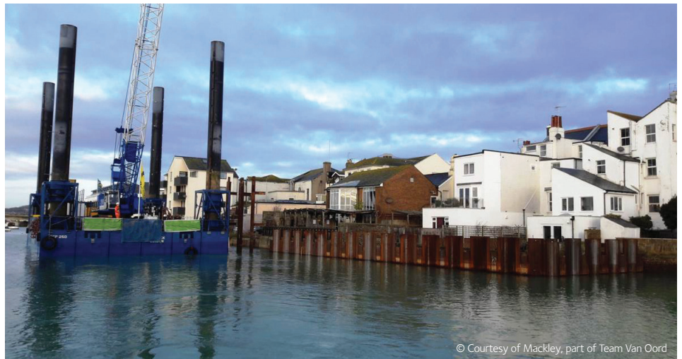
Reach E1: HZ/AZ installation from a jack-up barge
