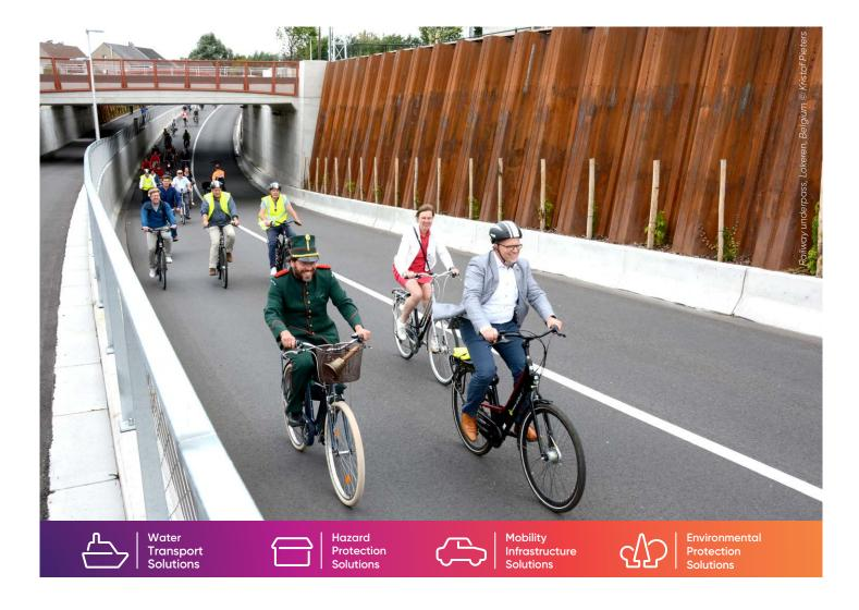
Steel sheet piles are widely used to form retaining walls for infrastructure projects, like ports and waterways or urban transport developments.
