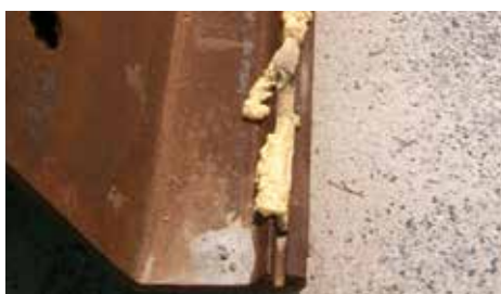
Closing interlocks with foam or grease
