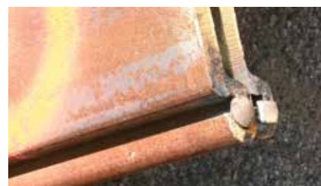
Bolt inserted in leading interlock
