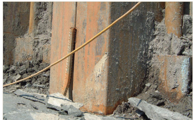
Pict. 1. Rock bolt on an AZ sheet pile
