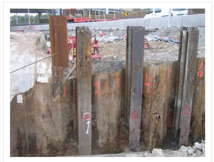
Pict. 4. H-beams with rock bolts supporting a steel sheet pile wall
