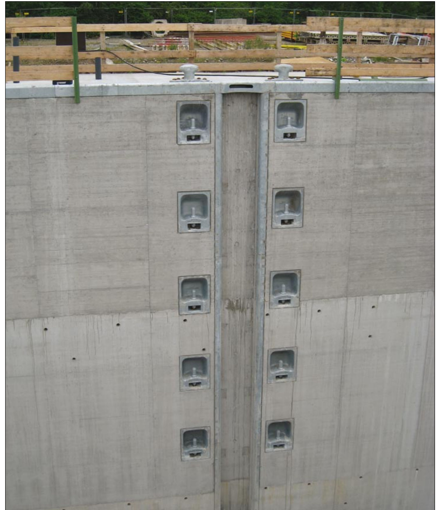
Baustelle Schleuse Münster Construction site of Münster lock
