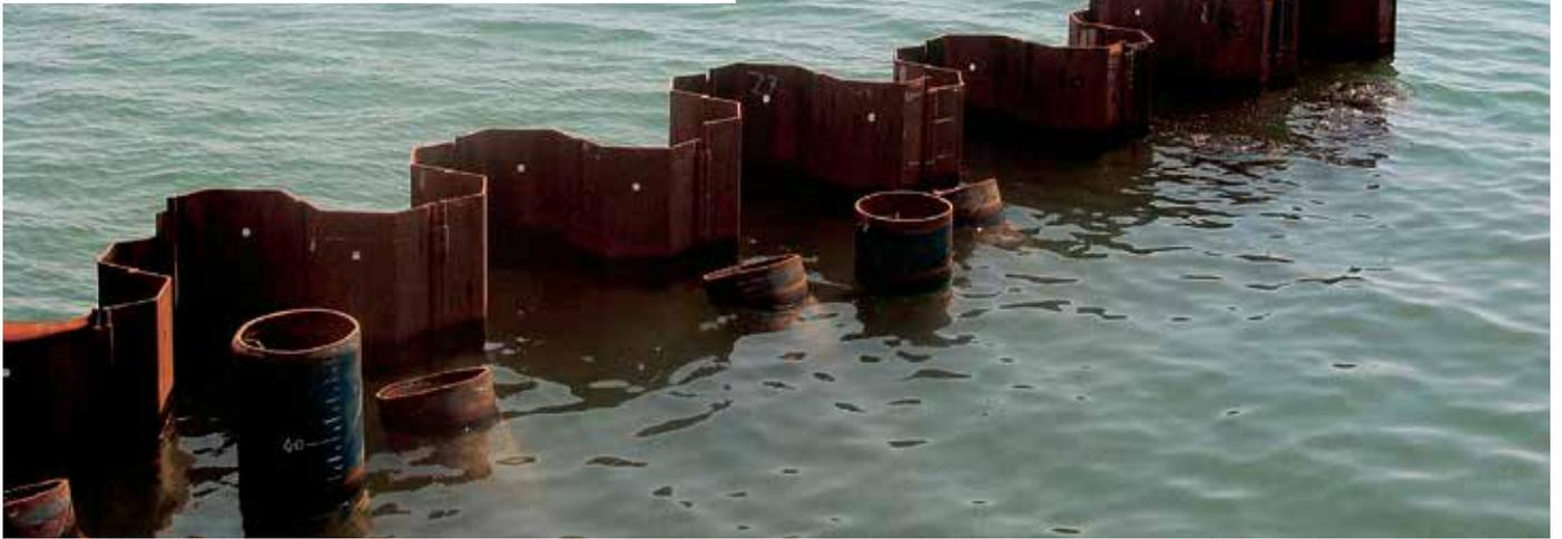
The structural system consisted of a sheet-pile soil-retaining wall, steel crane-foundation piles, and deflection-restricting batter piles.
