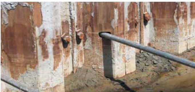
Tie rod/sheet pile wall connection details.
