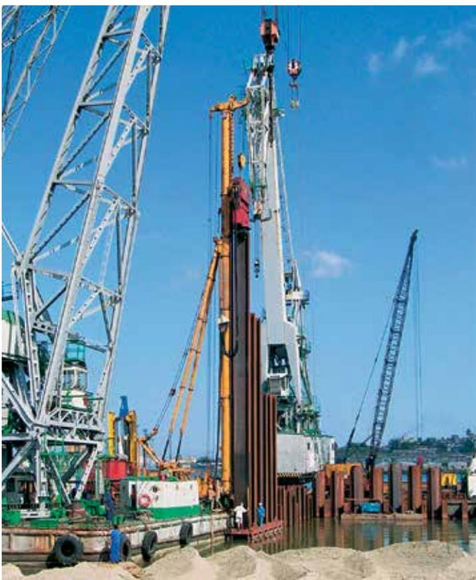
Several sheet piles were installed from a barge; others were driven with land-based equipment.
