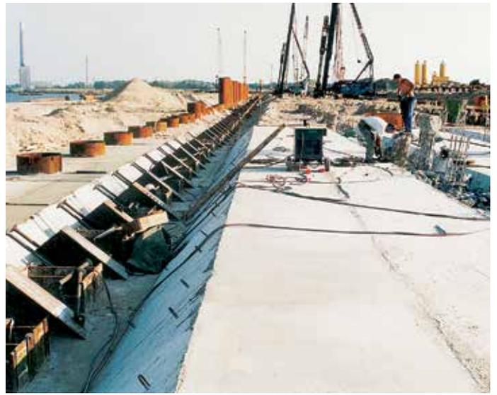
*After pouring, the concrete of the relieving platform was covered with a 3.3 m sand layer.*
