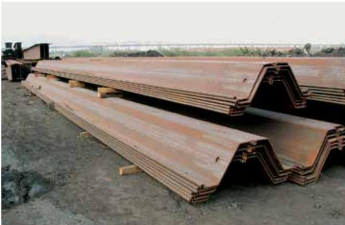
Wooden spacers prevent damage to the stored AZ piles.
