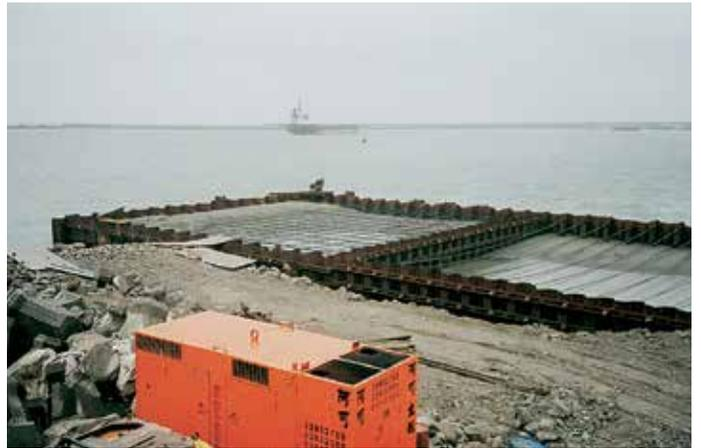
*The 27.4-m return wall of Quay 15 consists of a combined wall with 14 HZ king piles.*
