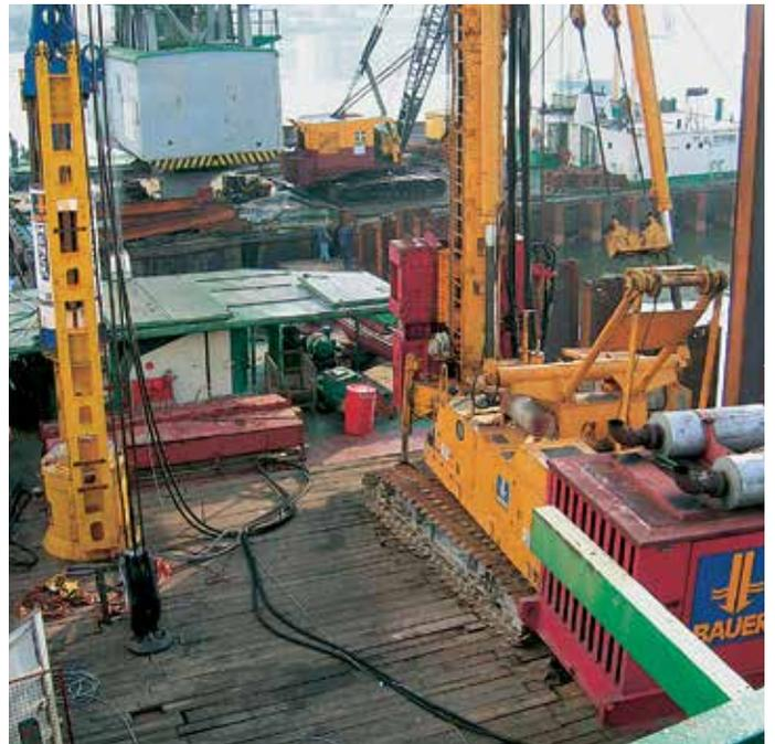
Bauer's pile-driving equipment: impact hammer and vibratory hammer.
