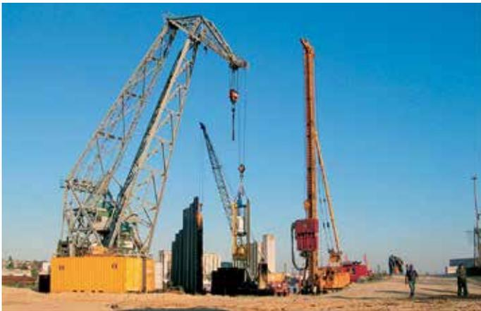
The HZ piles were driven by vibratory hammer until refusal, then taken down to design depth by impact driving.
