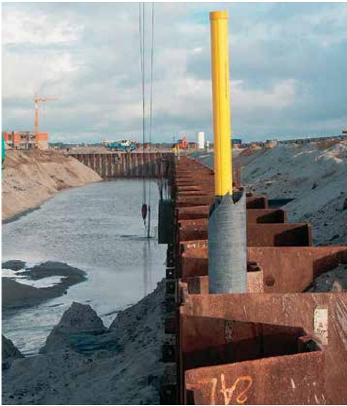
Dynamic bearing tests confirmed the vertical bearing capacity of 1,800 kN.
