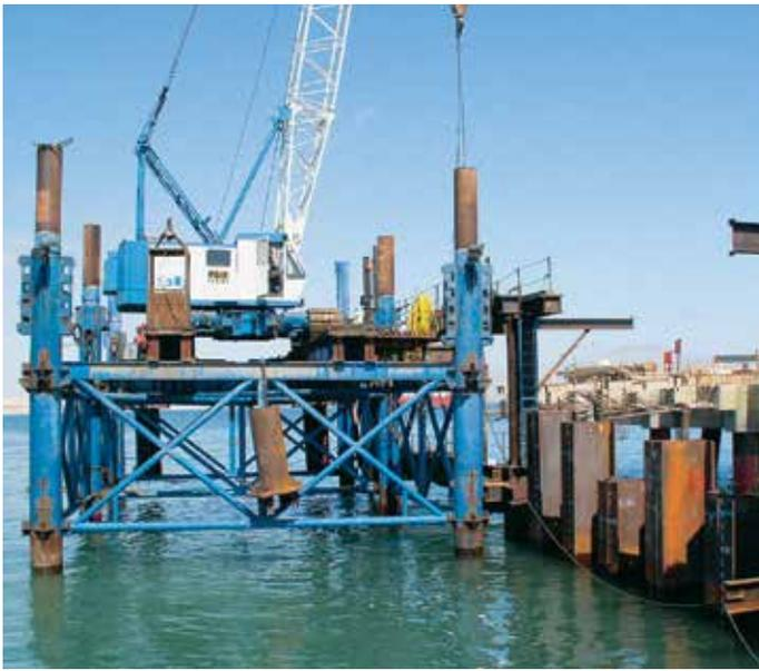
A jack-up barge and a template were used to install the HZ/AZ system.
