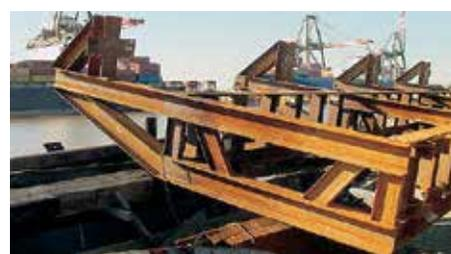
Neoprene shields attached to the template protected the coating system during installation.
