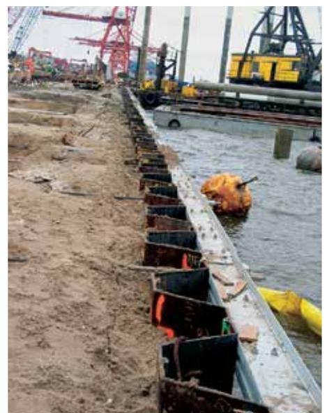
A waling system evenly distributes anchor forces into the sheet pile wall.
