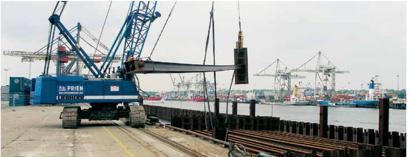
A crane lifted the preassembled anchors into position.
