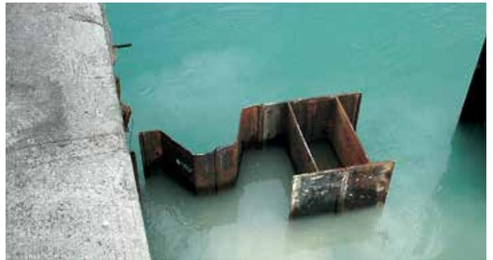
The connection between old and new quay consists of a steel plate welded to the first sheet pile.
