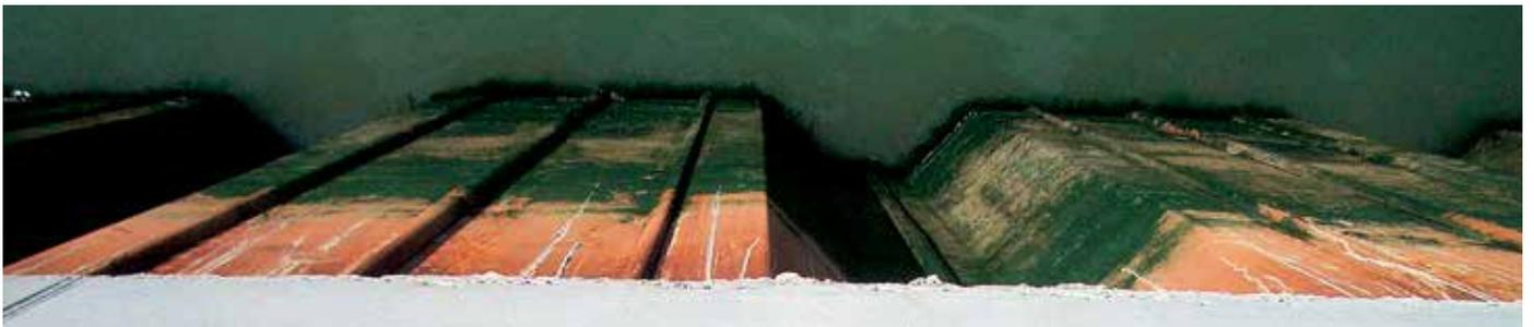
*HZ 775 C -26 / AZ 12 quay wall offering a water depth of 8.5 m.*
