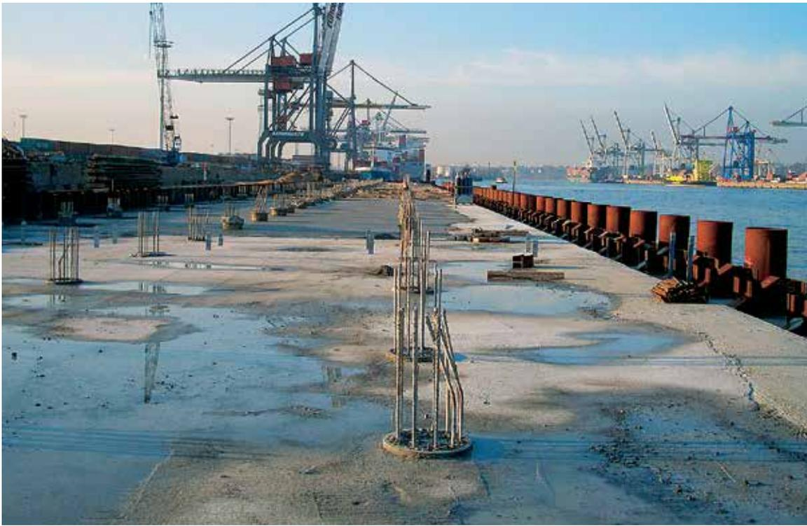
The structural elements of the quay comprise sheet piles, steel tubes, tension anchors, concrete columns, and the load relieving-superstructure.
