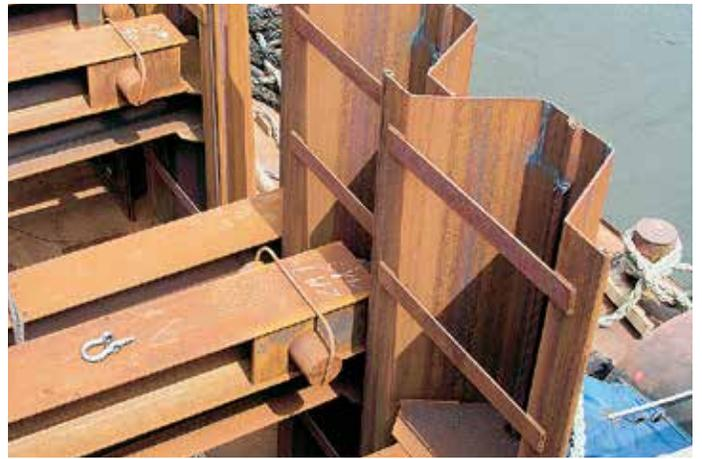
The 3.5 m AZ 25 piles transfer tensile forces into the backfilled soil
