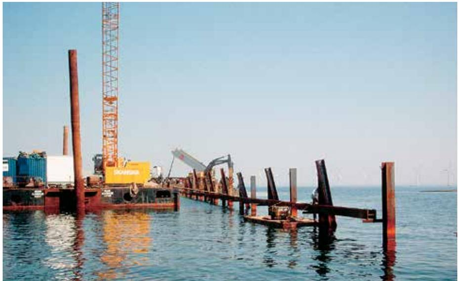
Horizontal beams were used as a driving template.
