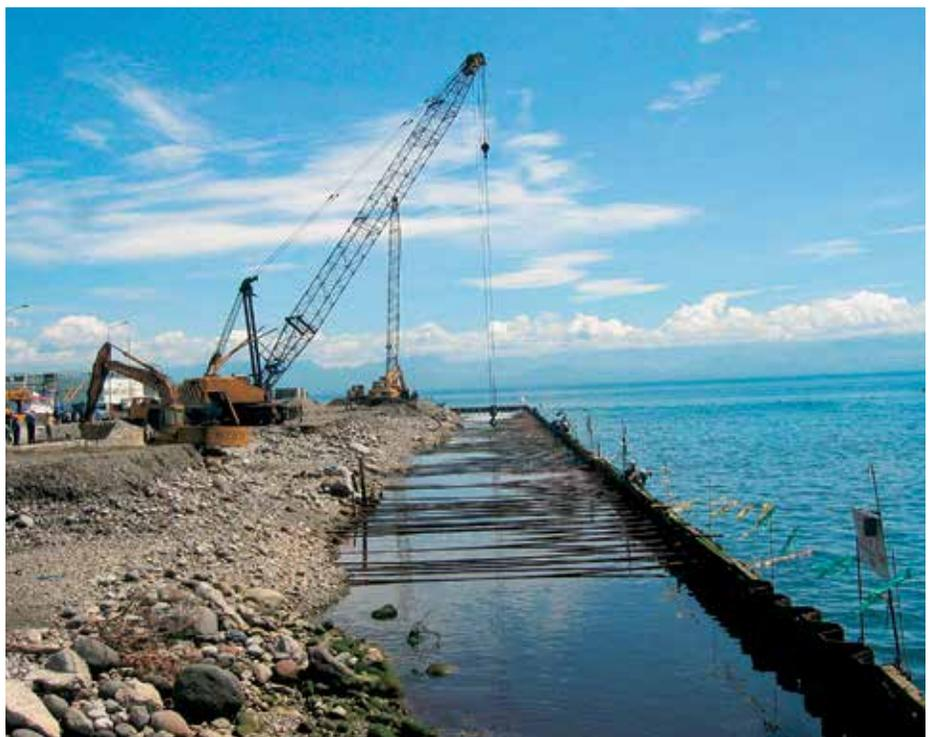
The new quay walls required 485 high-strength-steel tie rods.
