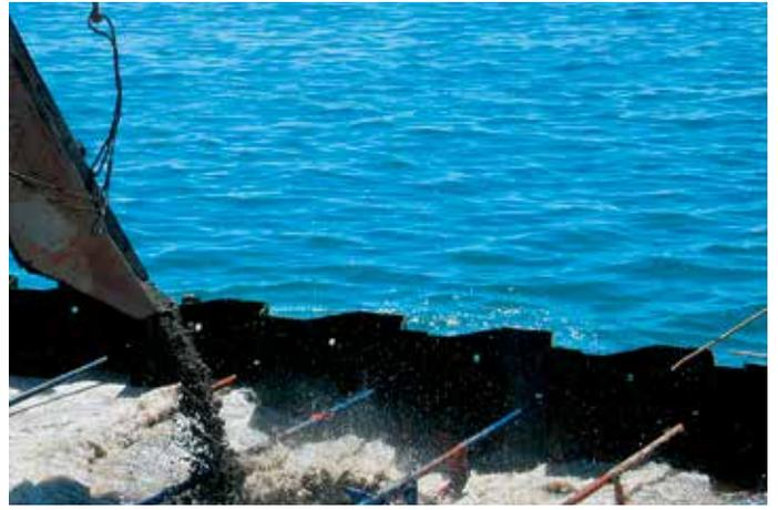
The area behind the AZ wall was backfilled carefully so as not to damage the tie rods.
