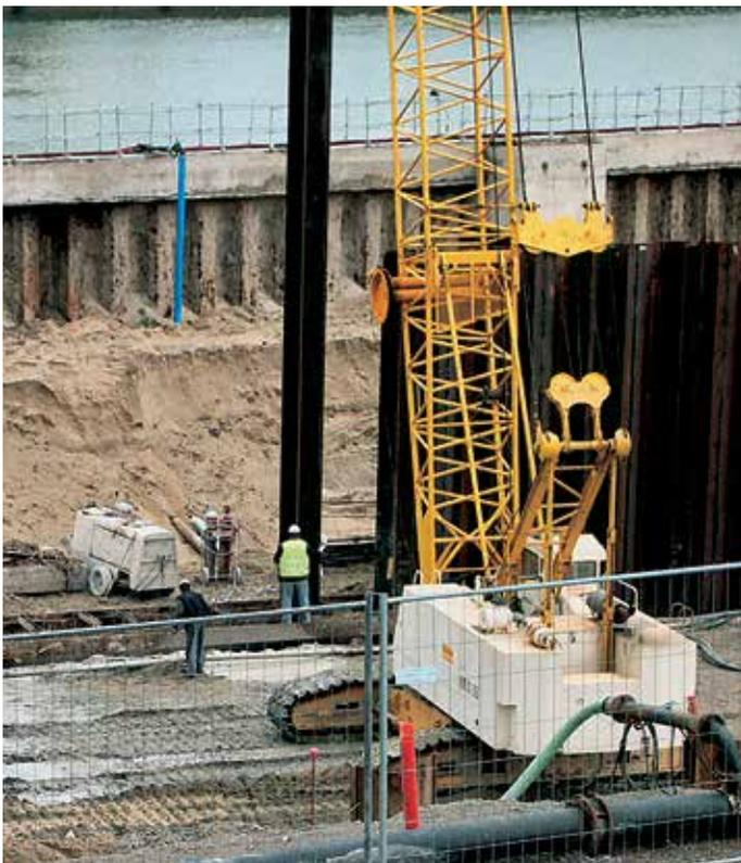
*A bentonite trench facilitated driving so that a simple template was sufficient.*
