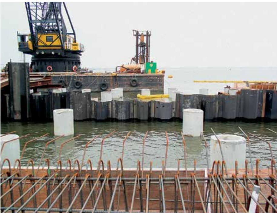
*The AZ 36 sheet piles take the static loads and act as an impervious water barrier.*
