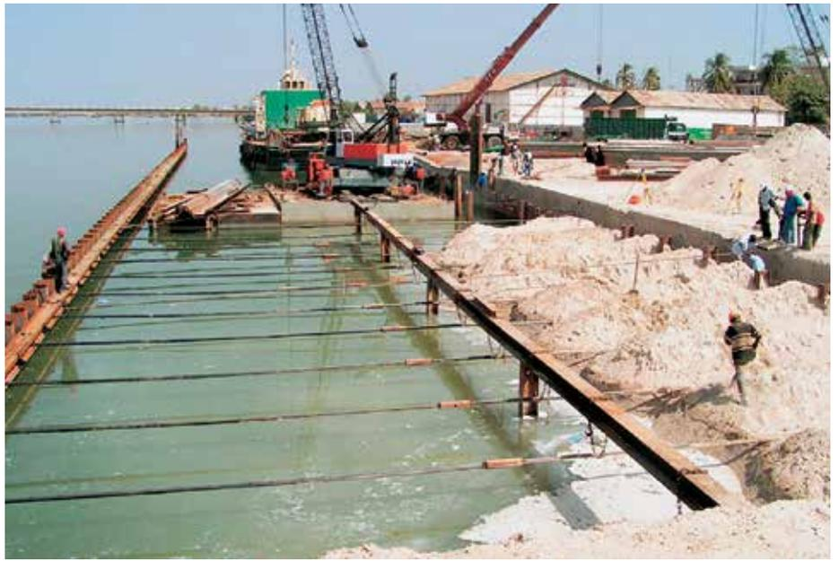
190 tie rods in different lengths were supplied by Anker Schroeder.
