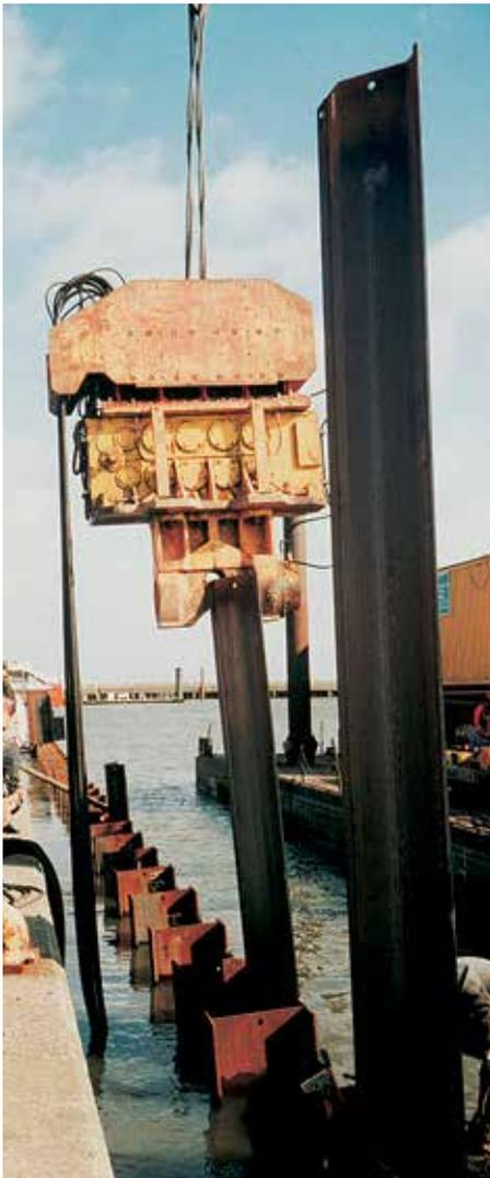
The vibratory hammer was the ideal tool to install the AZ intermediary sheet piles.
