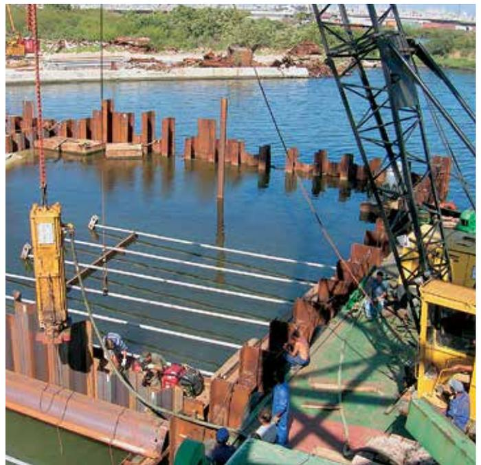
*Driving of steel sheet piles with barge-mounted equipment.*
