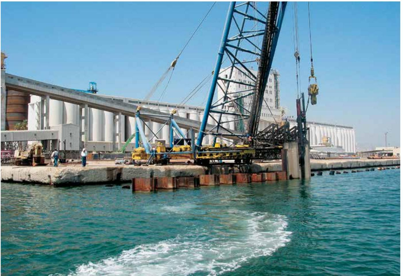
*The existing concrete structure was modernised with the help of a jagged sheet pile wall.*
