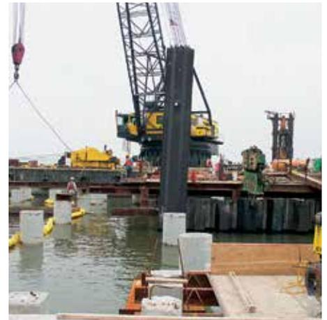
A template ensures the straightness of the sheet pile walls.
