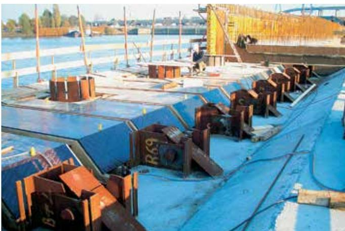
The load-relieving concrete superstructure installed at elevation +3 m provides for economical design of the combined sheet pile wall.
