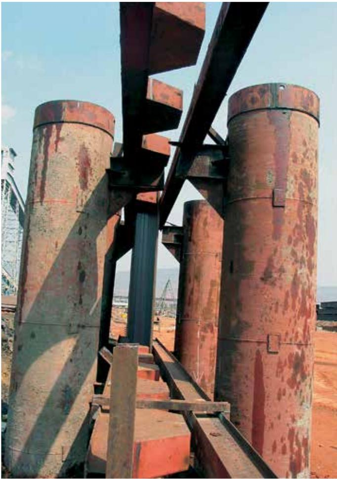
Two-level templates ensure correct horizontal and vertical positioning of the sheet piles.
