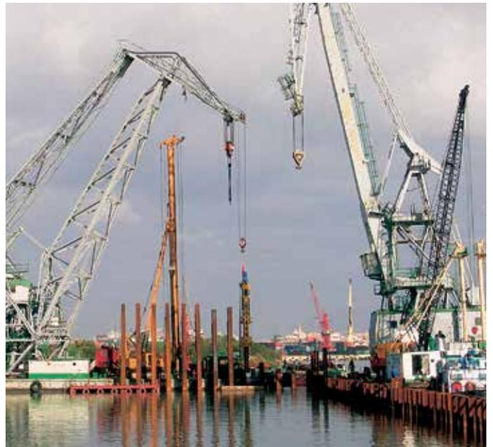
A locally hired floating crane assisted the installation of the combined sheet pile wall.
