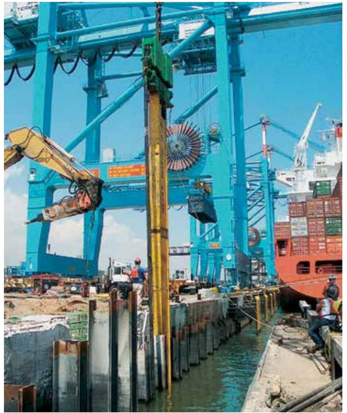
A special beam transmitted the vibration energy to the underwater AZ-piles.
