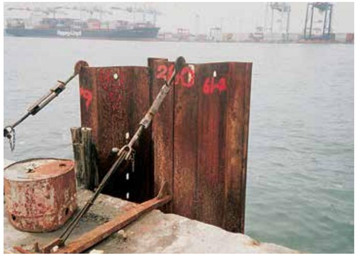
The piles were driven hard alongside the existing berths.
