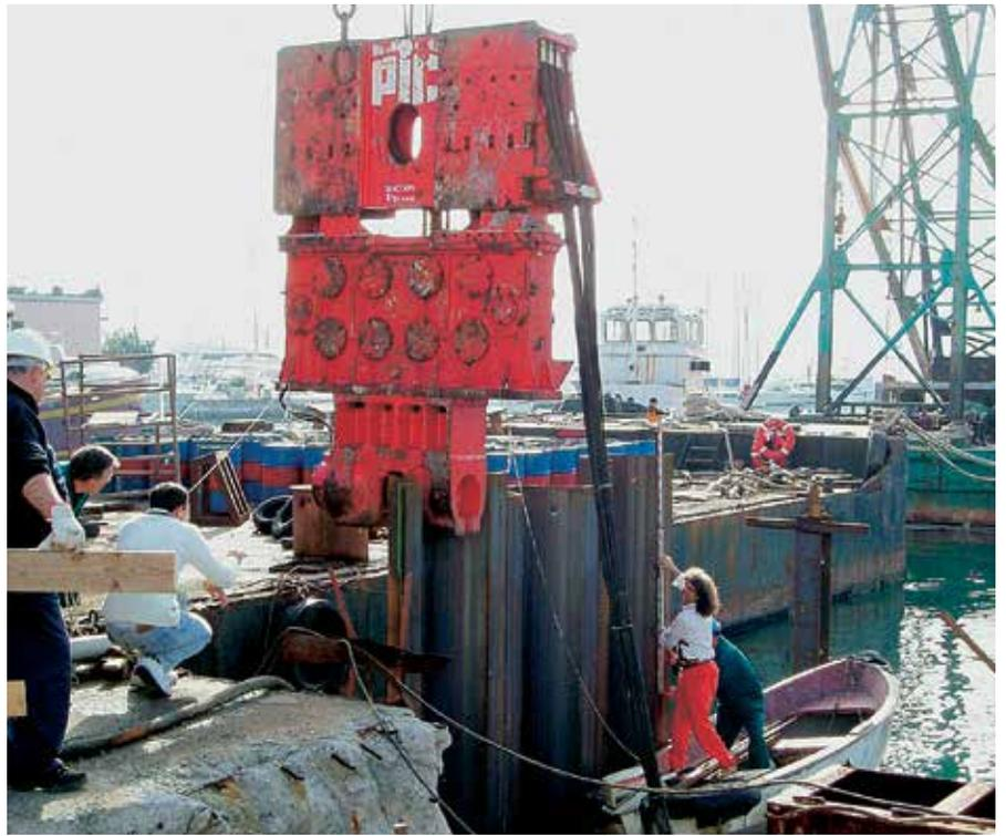
*Installation proceeded smoothly with the PTC vibratory hammer and the driving template.*
