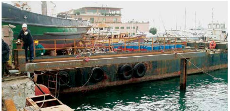
The new 400-m pier will be completed by 2006 using AZ 36 and AZ 18 sheet piles.
