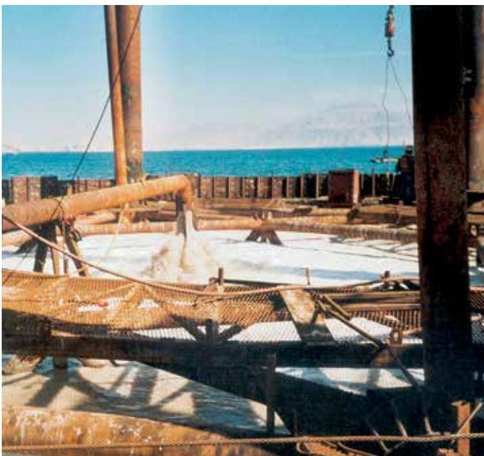
*Sheet pile cells are usually filled with locally available sand.*
