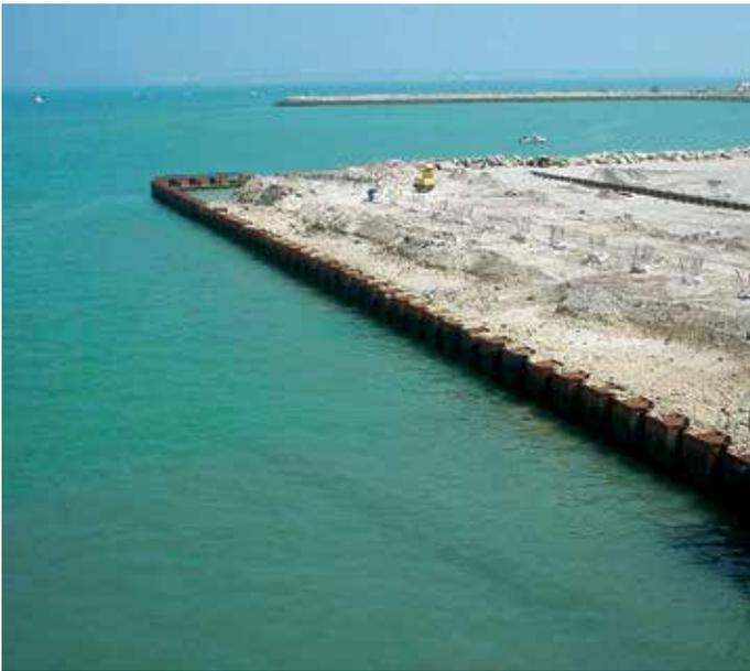
Once the sheet pile wall was installed, the area behind it was backfilled.
