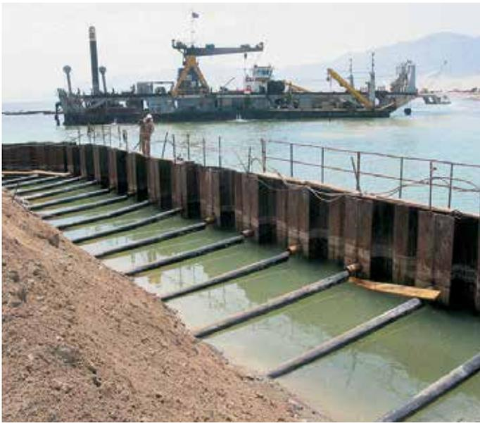
An anchored combined sheet pile wall was chosen as the optimum solution for the quay wall.
