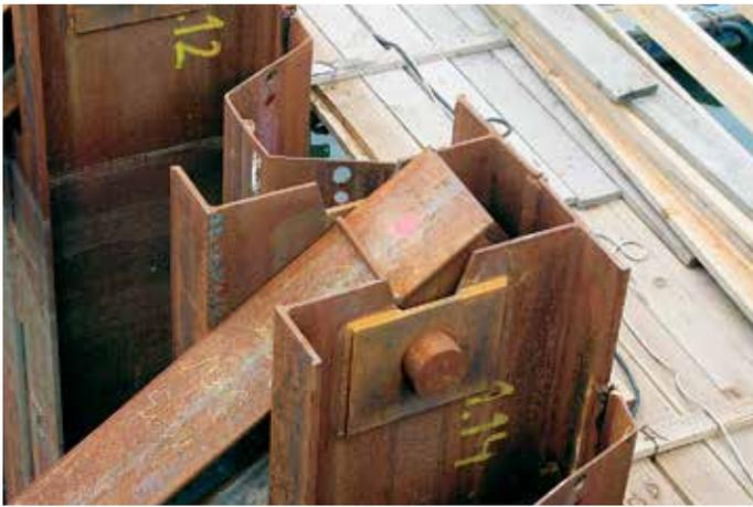
A 170-mm-diameter pin forms the pivot of the anchor system
