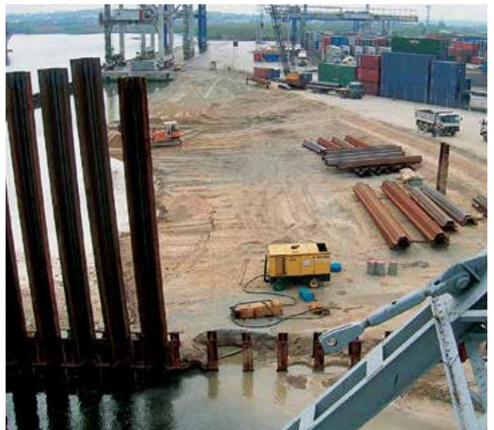
The AZ piles were inserted between the HZ piles then driven to design depth.
