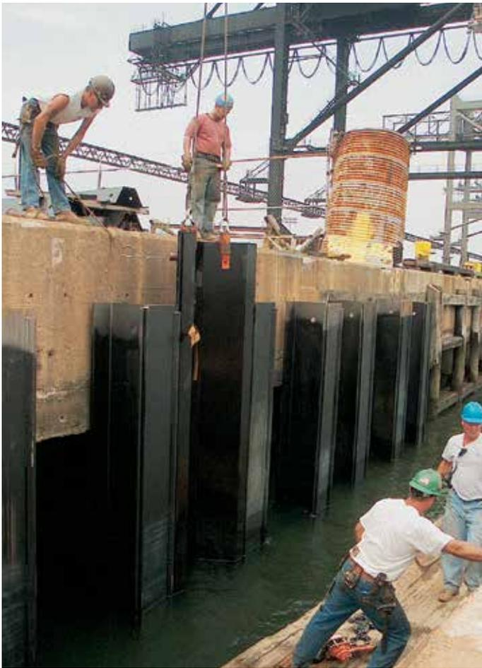
The heads of the HZ king piles remained above the water line, which facilitated their installation...
