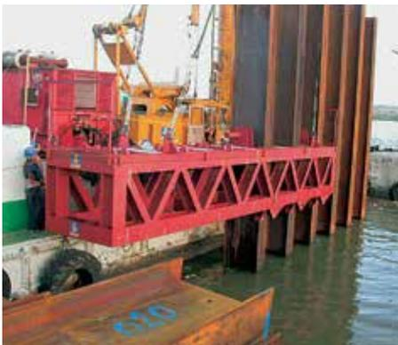
Precise positioning of the HZ king piles was guaranteed using a double-level template.
