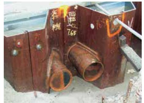
A hole was cut into the piles to pass the rebar tie rods.
