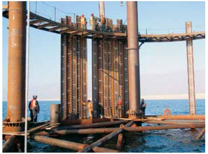
The straight-web sections were installed with the help of a template to form the breakwater cells.
