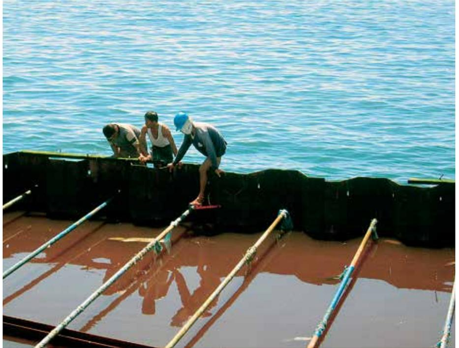
The tie rods consisted of several parts suitable for transportation in 40-foot containers.
