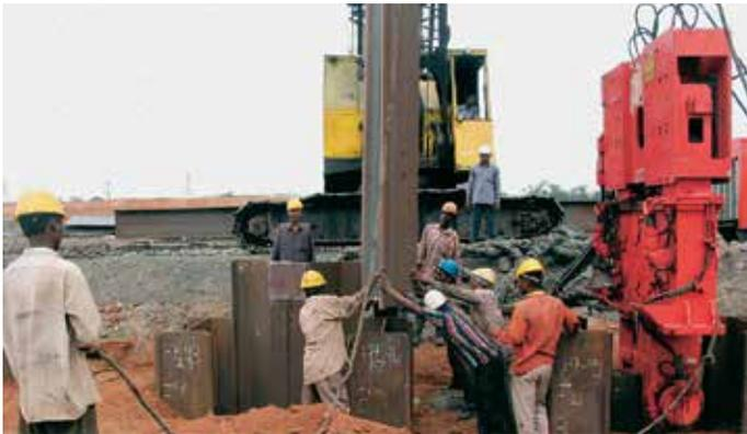
Due to the presence of weathered rock an impact hammer was needed to fully drive the sheet piles.
