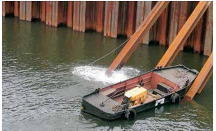
At an angle of 32°, the vibratory hammer was switched on to securely position the anchor.
