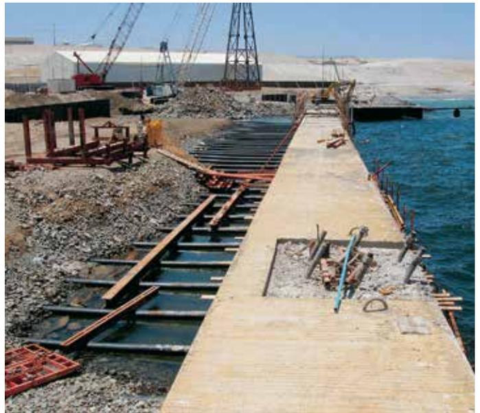
A concrete capping beam supports fenders and bollards.
