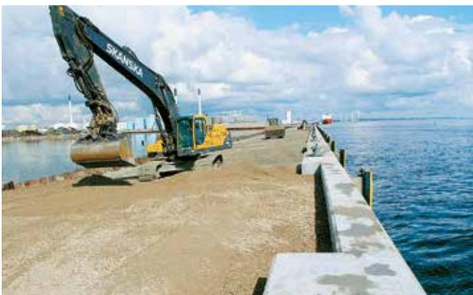
*A capping beam fitted with fenders and bollards was placed on top of the sheet piles to finish off the construction.*
