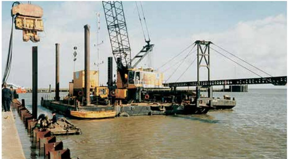
After installation of all the king piles, the AZ sheet piles were driven to El. -20 m.
