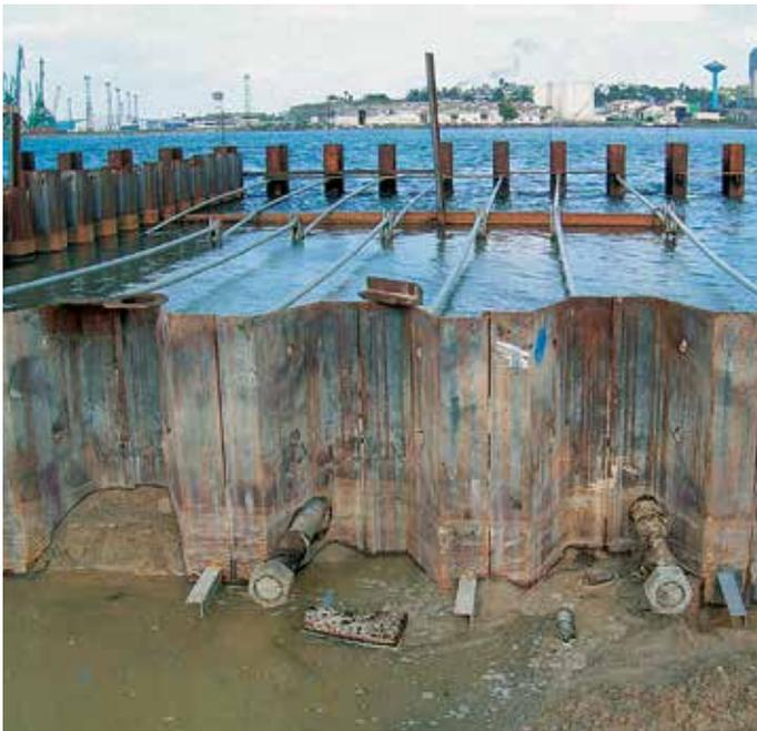
The complete solution provided includes front wall, tie rods, and anchor wall.
