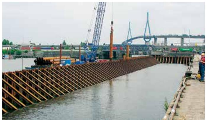
The new sheet pile wall of Berth 1 was placed 36.9 m in front of the old quay wall.
