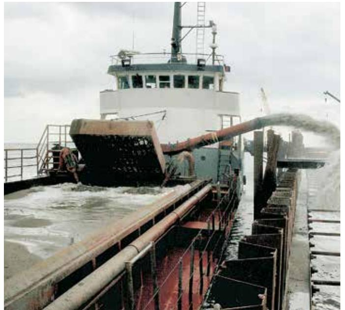
*The cofferdam was filled with dredged sand.*
