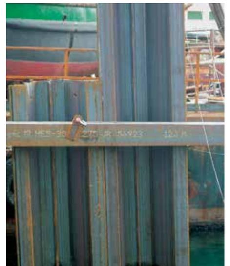
A template was used for the installation of the AZ piles.
