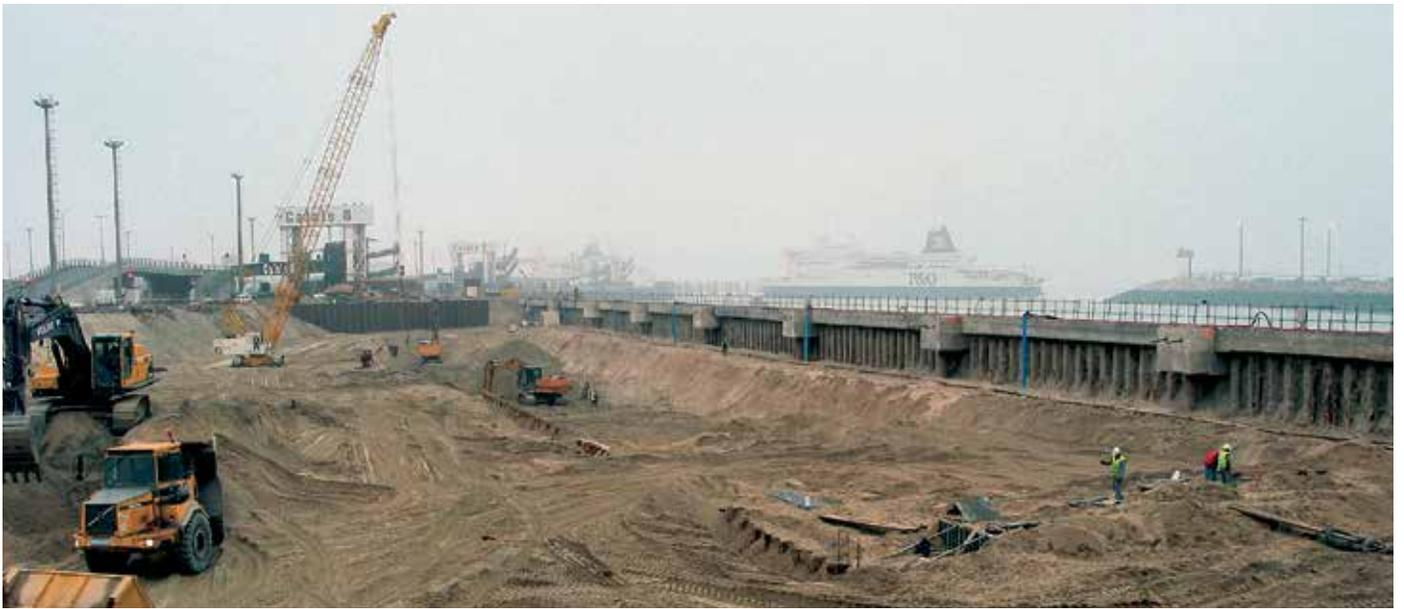
The existing PU 25 quay wall allowed the new wall to be driven in the dry.
