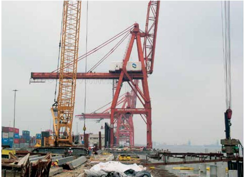
*Installation by land-based crane equipped with vibratory hammer.*
