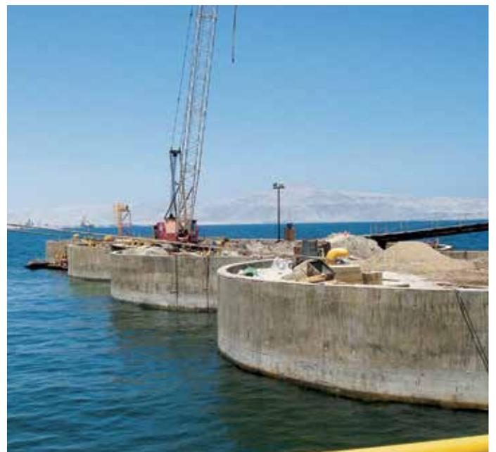
*Concrete ring beams protect the cells.*
