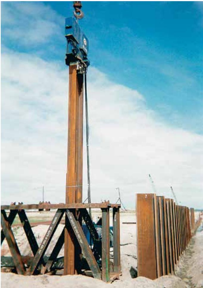
*A two-level-template ensured straightness during installation.*
