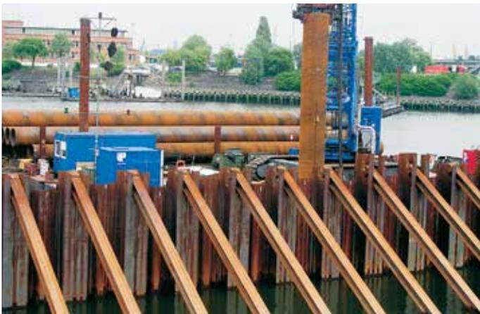
Steel tubes take vertical loads and minimise scouring.
