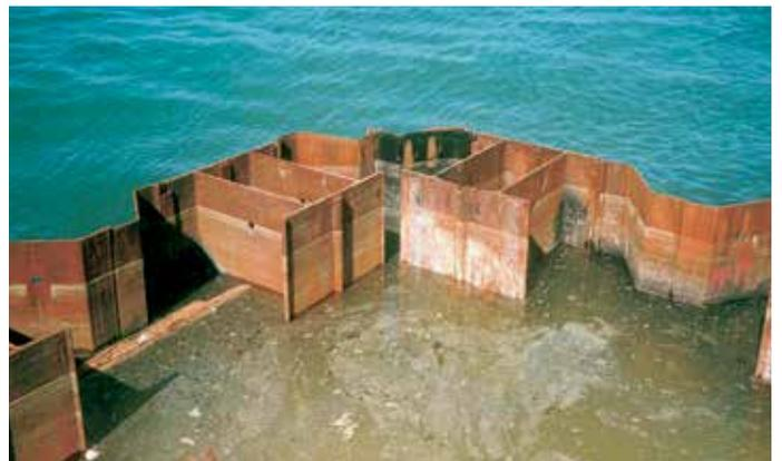
The wall's corner consists of AZ 18 piles that were also used as intermediary piles.
