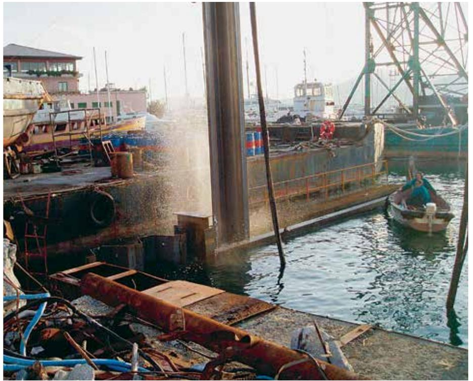
2,600 t of 24-m AZ 36 and 8-m AZ 18 sheet piles were installed.
