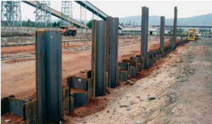
The Indian designer Howe opted for an anchored HZ/AZ combined sheet pile quay wall.
