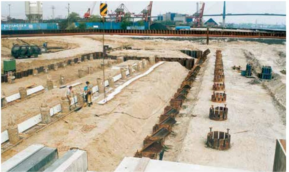
The low-level superstructure slab is placed on top of the two sheet pile walls, steel tension piles, fender tubes & concrete piles.
