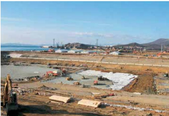
*A dry dock for offshore platforms was built using more than 3,000 metric tons of steel sheet piles.*
