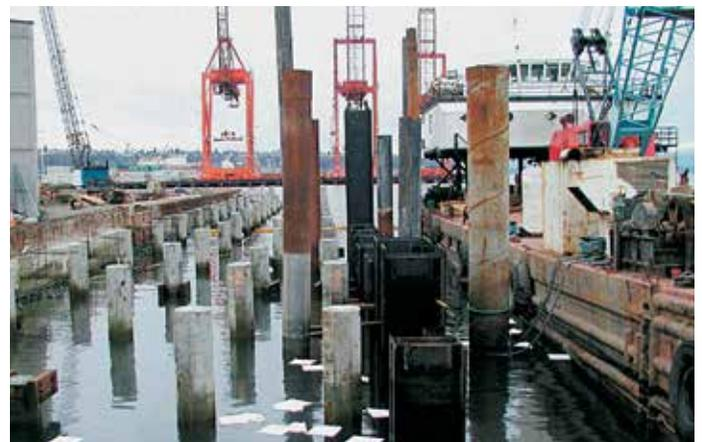
The steel sheet pile wall that stabilised the structure was installed from a barge.
