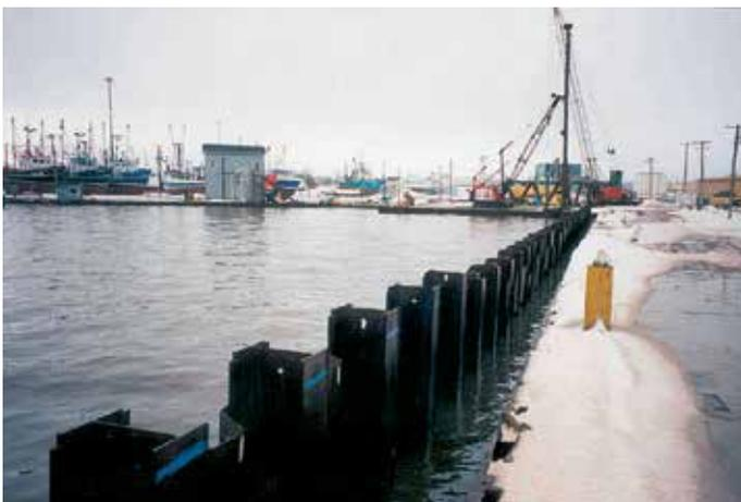
New sheet pile wall installed 1.5 m in front of the existing wall.
