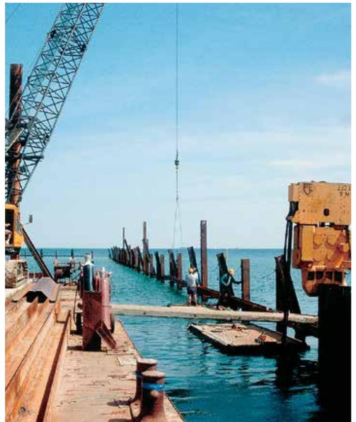
*The crane, vibratory hammer and sheet piles were loaded on a barge.*
