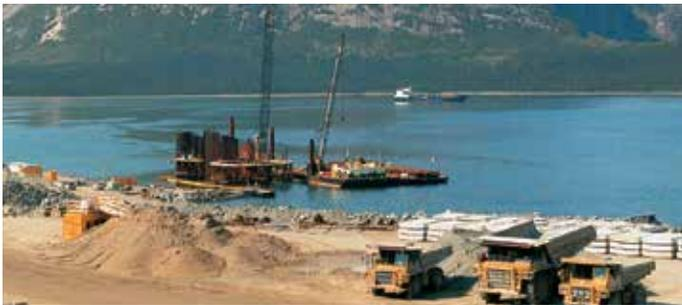
Piles were driven with barge-mounted equipment.
