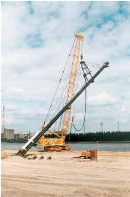
The 47-m tailor-made HTM 600/136 anchor piles were driven with a hydraulic impact hammer.
