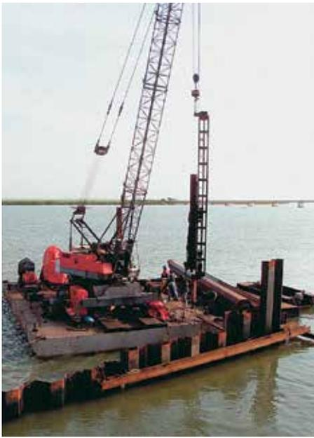
Delmag diesel impact hammer.
