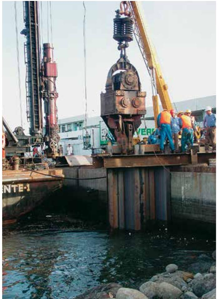
*A vibratory hammer was used first; a diesel hammer then completed the installation process.*
