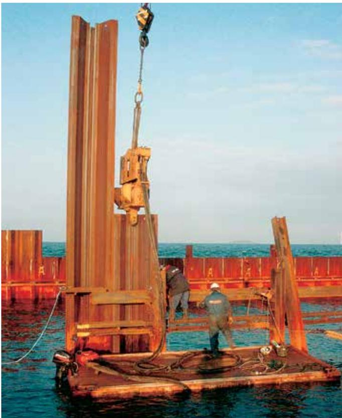
*Several barges facilitated the installation of the two cofferdam walls.*
