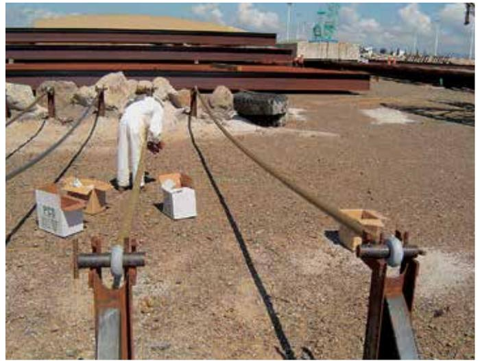
Corrosion-protection tape was wrapped around the anchors.
