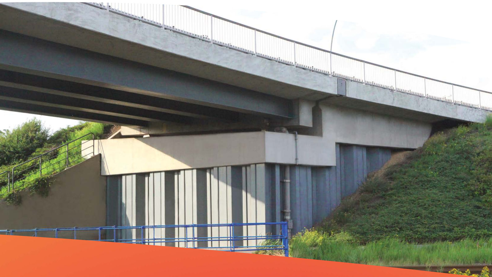
Fig. 3. Example of a conventional road bridge abutment using combined sheet pile walls (high stiffness) and discrete bearings (Hamburg, Germany).
