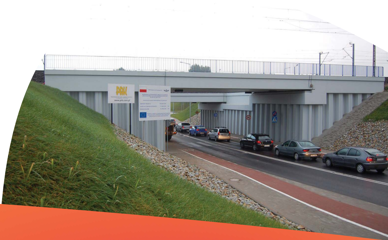
Fig. 1. Steel sheet pile (ca. 300 t of AZ 50) bridge abutment (Swarzędz, Poland).
