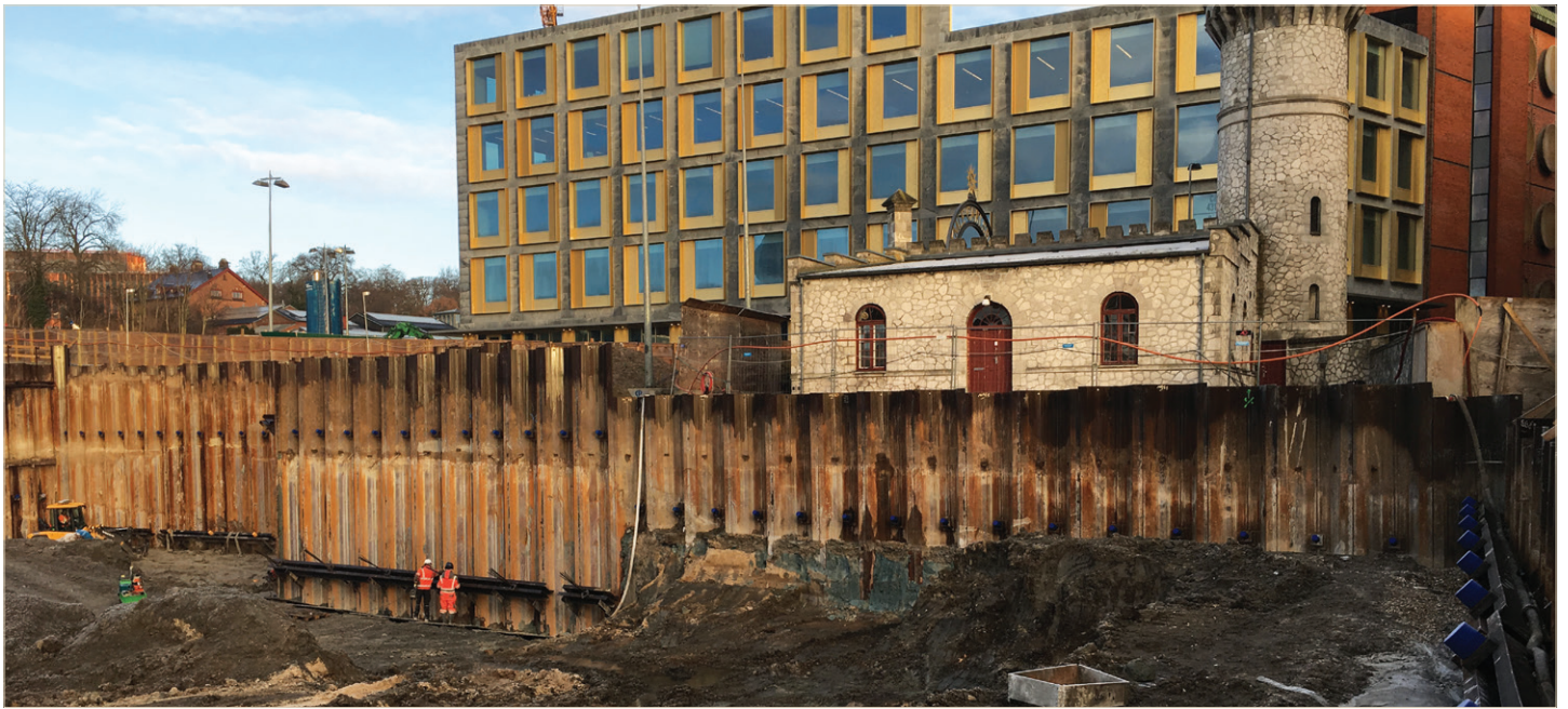
Fig. 27 – Retaining wall with 2 anchor levels.
