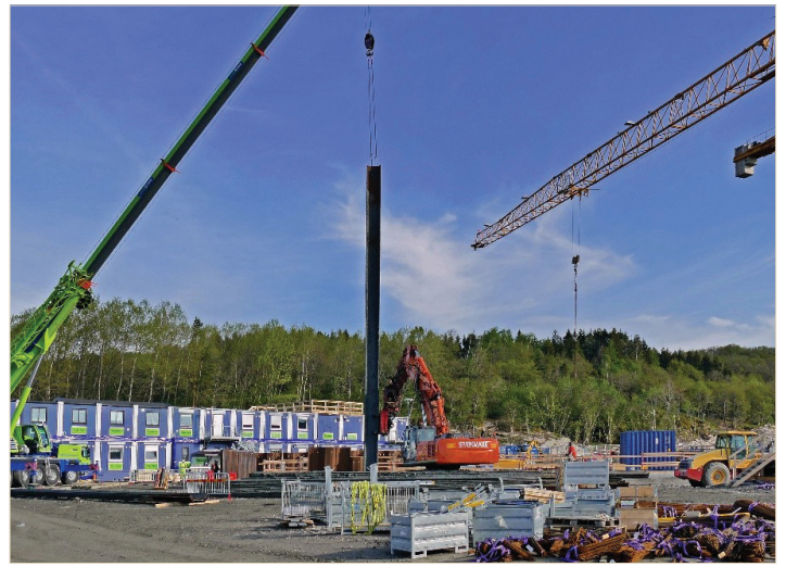
Fig. 7 – Extraction of the sheet piles ongoing for building 16.
