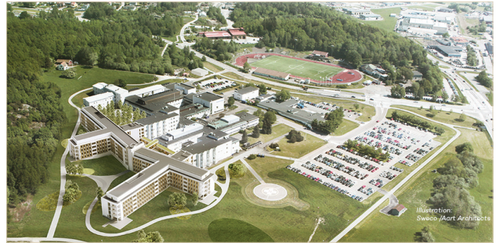
Fig. 1 – Aerial view of Kungälv Hospital (© Skanska – Sweco).
