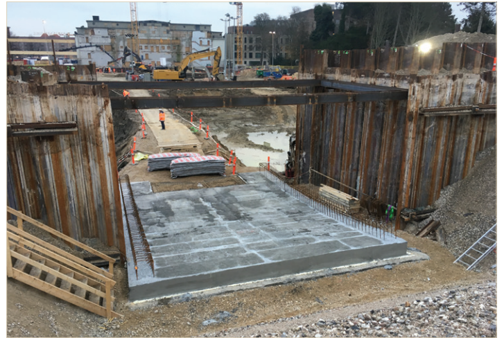
Fig. 29 – Detail of one of the retaining walls.
