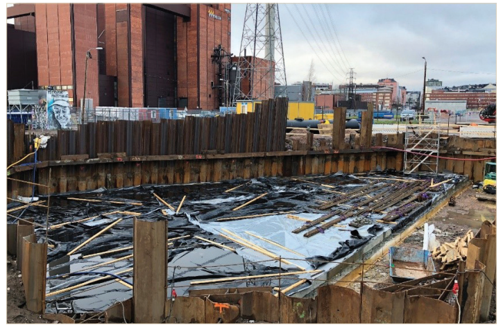
Fig. 35– Execution of the cofferdam.
