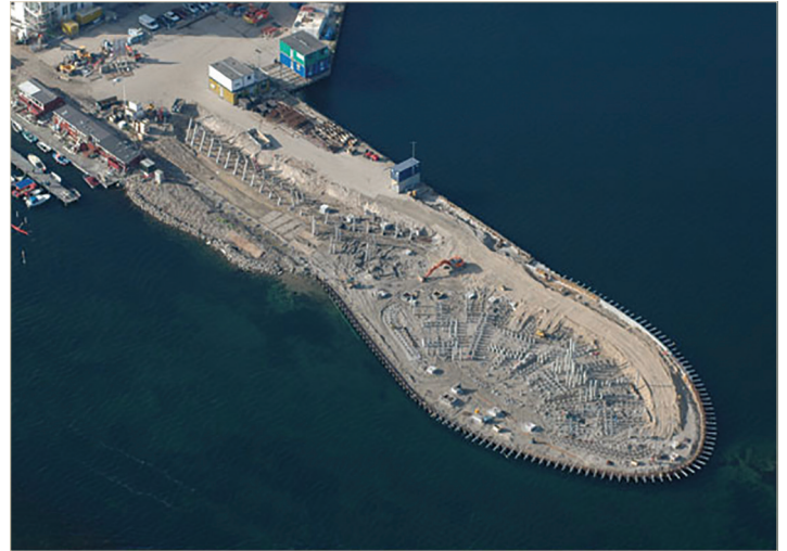
Fig. 30 – Aerial view of the construction site.
