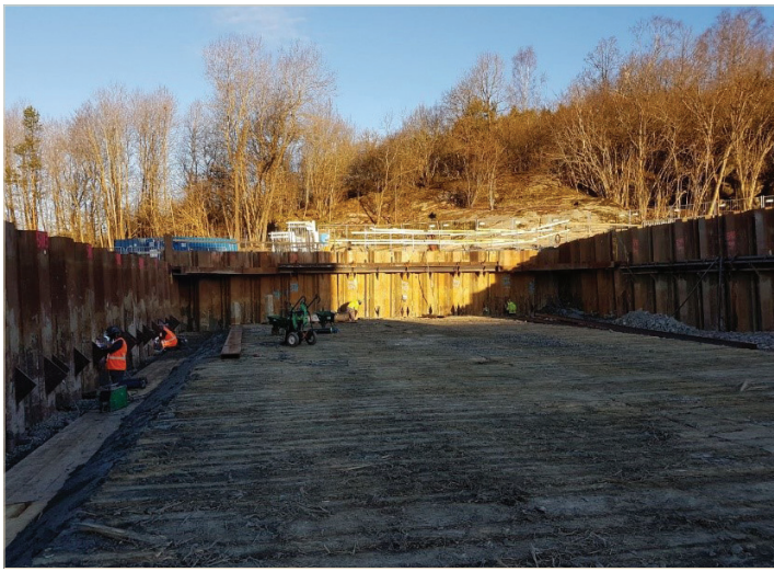
Fig. 4 – Welding of a waling on the sheet piles for building 17.
