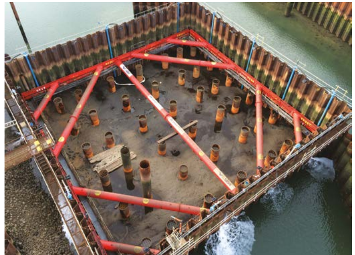
Photo: Ipswich tidal barrier, UK | ©MGF
