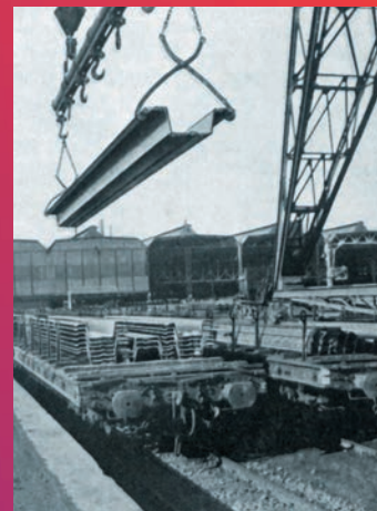
Belval steel works, Luxembourg, 1930s
