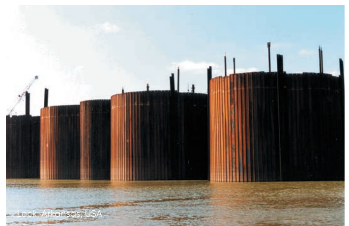
Diaphragm cells with 120^\circ junction piles.
